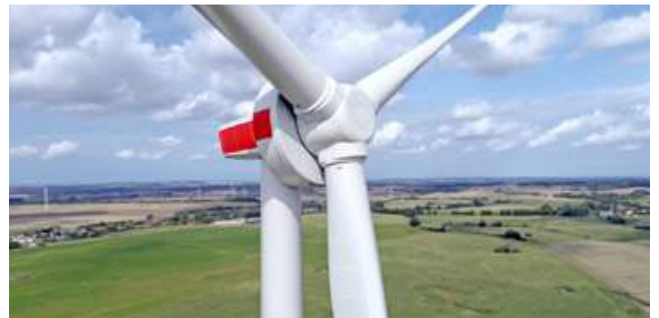
HYGRO specialises in the production, delivery and distribution of hydrogen produced directly from wind. It is building a 4-MW wind turbine with an integrated electrolyser in the province of North Holland. The aim is to maximise synergy between wind power, hydrogen and pipeline & storage technology. The concept optimises conversion of wind power to hydrogen, which can be transported at much lower cost than electricity and with a significantly lower impact on spatial planning.
