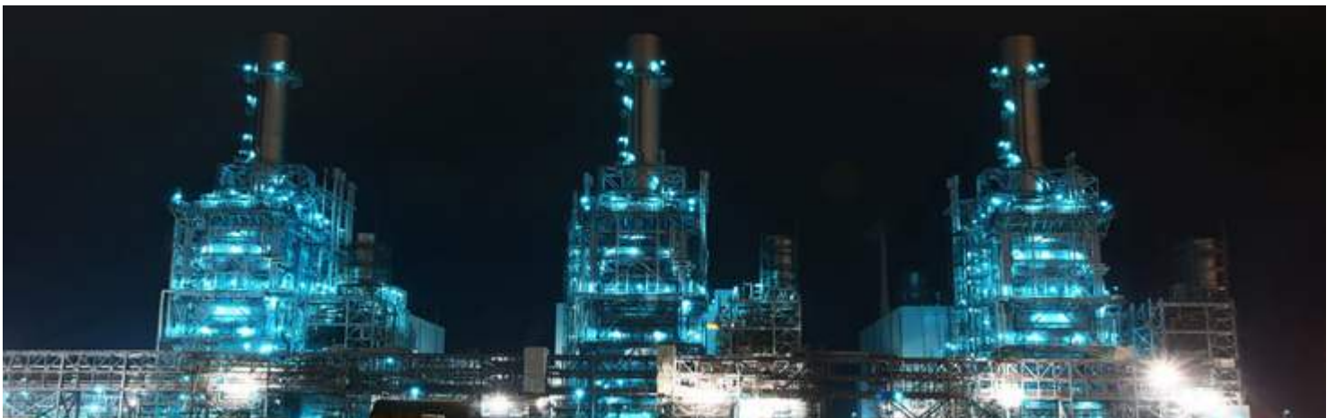
In the Eemshaven, the port in the north of the Netherlands an existing gas-fired power plant is being prepared to convert to hydrogen. After acquiring the plant from Vattenfall in 2022, RWE continues to pursue the ambition of having the first of the plant's three 440-MW units run on (low-carbon) hydrogen by 2025. By converting the remaining units and switching to clean hydrogen by 2030, this is likely to become the world's first carbon-neutral hydrogen-fuelled power plant.
